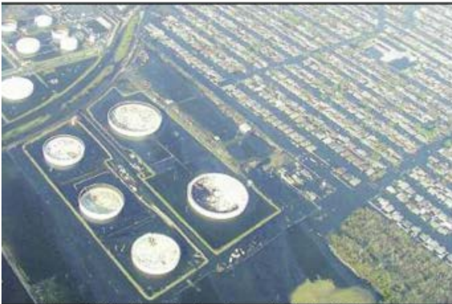
Figure 1: Oil leaks from hurricane-damaged oil tanks. USCG photo.
