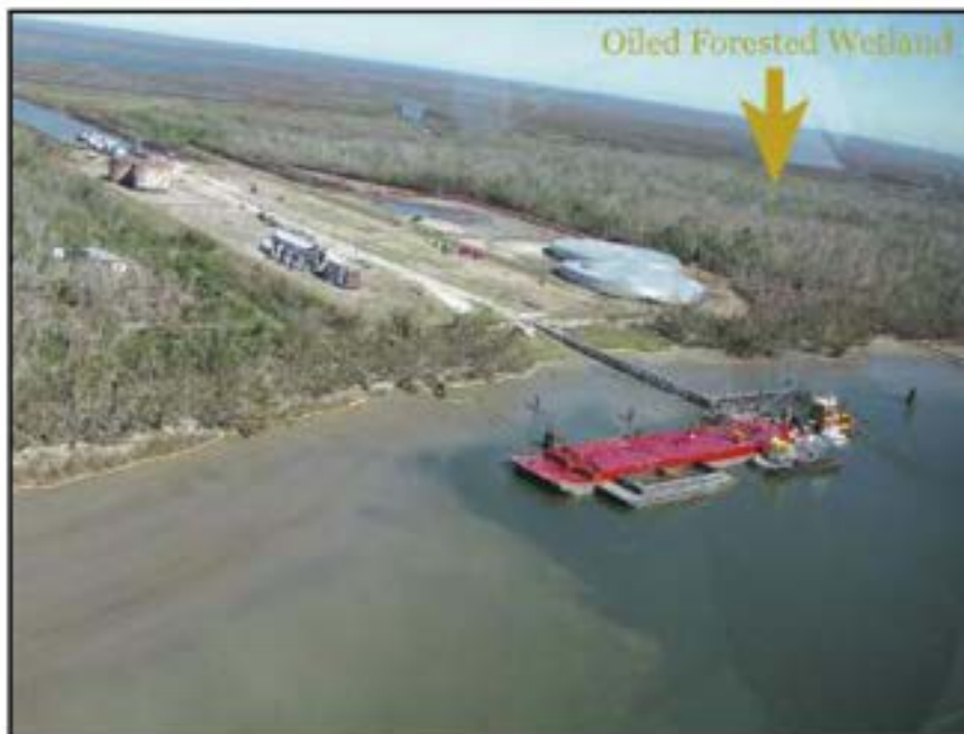
Figure 2: Oil from damaged tanks was moved by hurricane forces into impassable forested wetlands. USCG photo.
